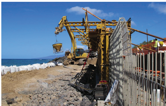
Fig. 3.2f—Construction of seawall with GFRP bars.
